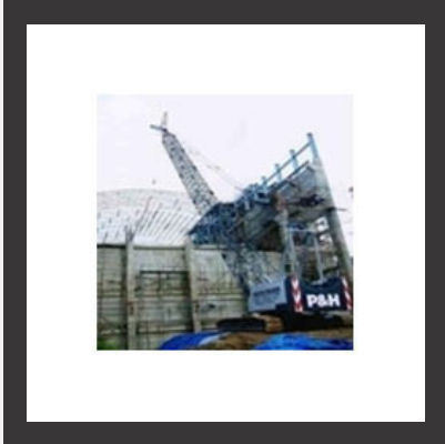
P & H Kobelco Crawler Crane Services
